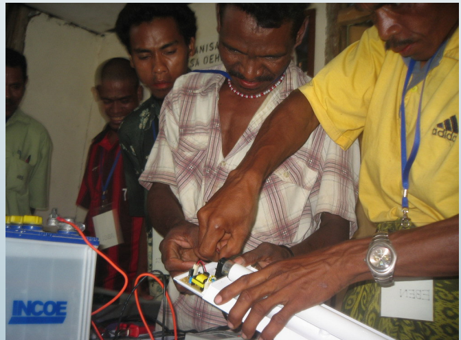
Installation of the inverter on the lamp Credits : YBUL
